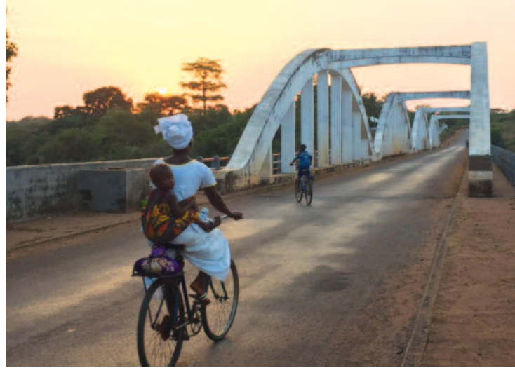
Photo: Mafalda Marchioro/UNDP Saltinho Bridge, Guinea-Bissau.
