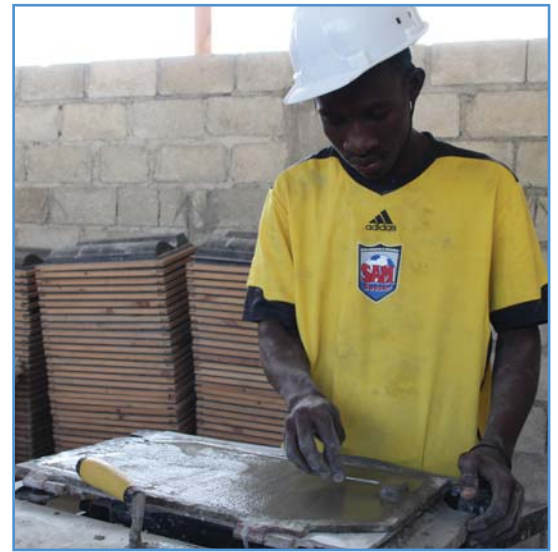
A worker is crafting a roof tile made from recycled debris, Carrefour-Feuilles, Port-au-Prince © UNDP-Haiti, 2012
