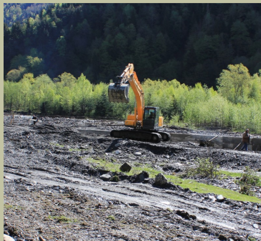
Photo 7: Construction of a protective dyke - Tsana 1
