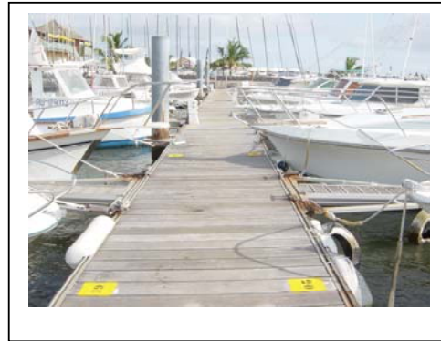
Floating docks for boat mooring
