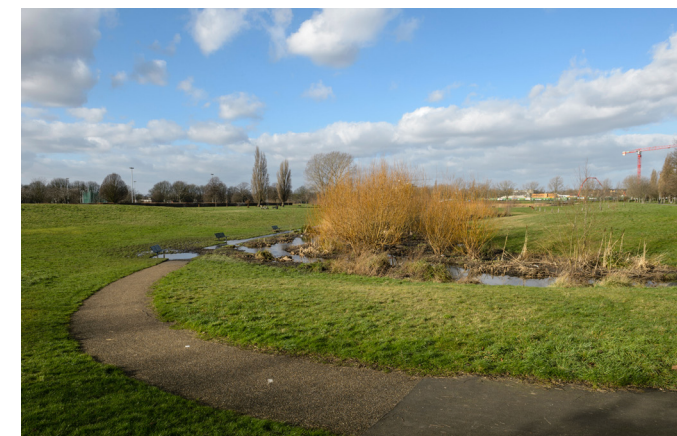
Figure 12: Sutcliffe Park in London - engineered landscape forming water impoundments. River Quaggy flood alleviation scheme.
