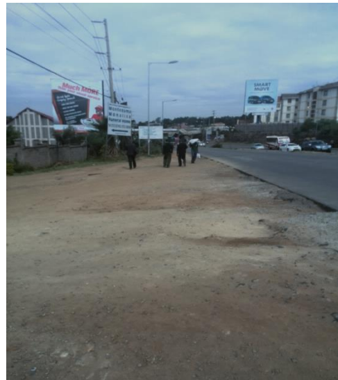
Figure 3: Pedestrian Walkway along Mbagathi Road, 2015
