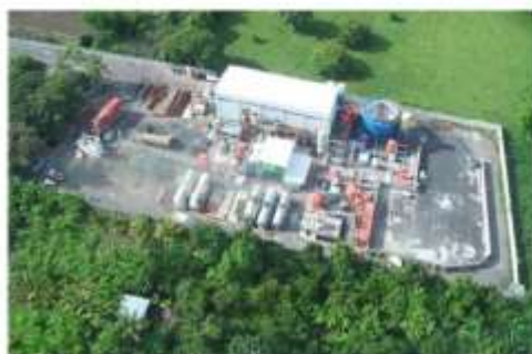
Source: Recovering S.A.
