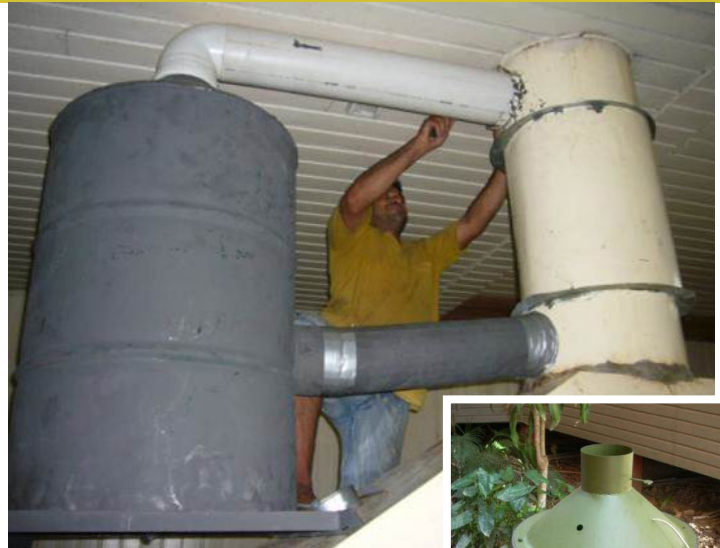
Above: The Mercury Capture System, shown being installed in a gold shop in Peru, can reduce mercury emissions by as much as 80%. Right: A prototype of the MCS before being field tested by the U.S. EPA and National Argonne Laboratory. Photos courtesy of the U.S. EPA.
