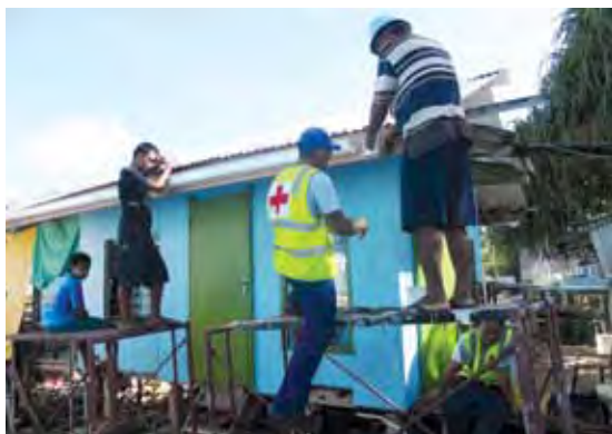
Repairing water infrastructure on Tuvalu.
