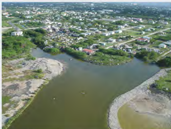
McKinnon's Pond, Antigua Demo site
