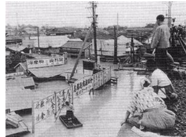
Levee break (top) and flooding (bottom), Tone River, Sep., 1944
