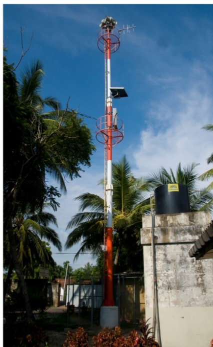
An example of part of an early warning system: 1 of 52 broadcast towers installed in Sri Lanka. ESCAP Photo.
