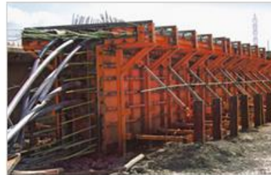
Flyovers at Santacruz airport Junction on Western Express Highway
