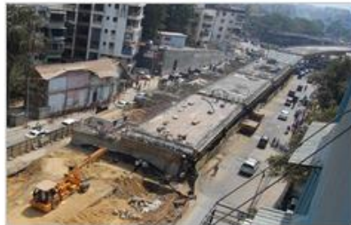
Flyovers at Barfiwala Lane Junction, Andheri
