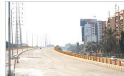
Flyover at Thakur Complex junction, Kandivali on Western Express Highway.
