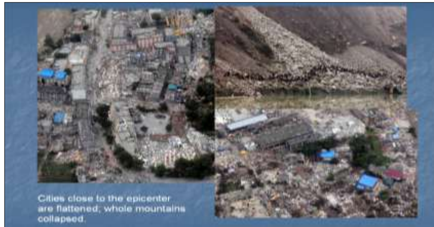
Wenchuan Earthquake, 2008, M8.0
