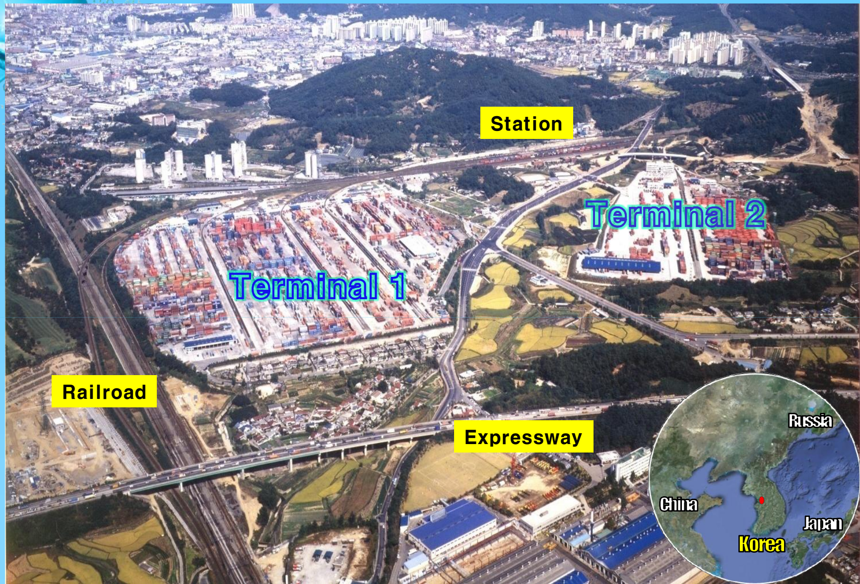
Uiwang Inland Container Depot
