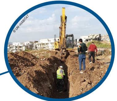
Installation of water pipes in Duhok
