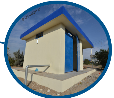
Construction of a new water well in Erbil
