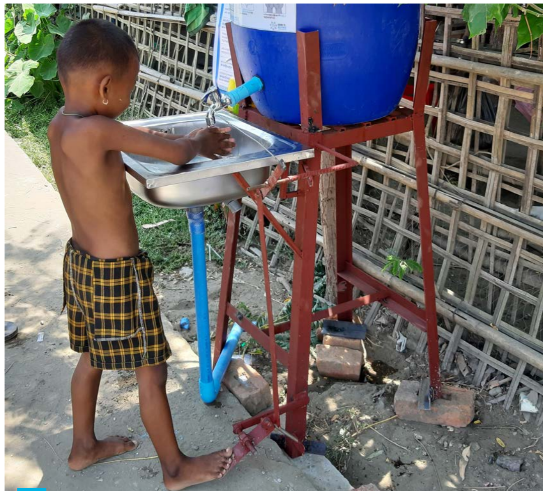
A child using a touchless handwashing facility installed by UN-Habitat that aims to prevent the spread of COVID-19 in Sittwe, Myanmar © UN-Habitat
