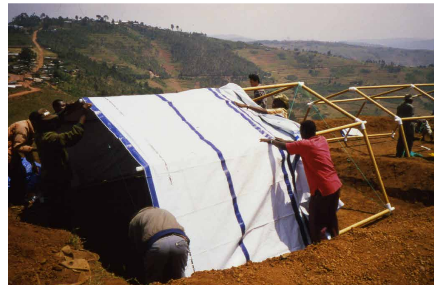
Shelters made of PT and tarpaulin under construction. Byumba Refugee Camp, Rwanda. Feb.1999. © VAN
