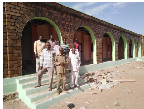
The new administrative building in Shangili Tobay using stabilised soil block (SSB)
