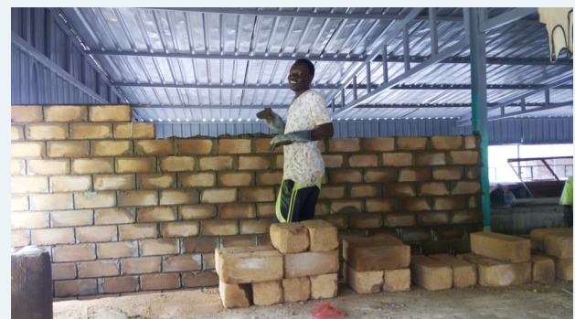
Trained youth engaged in construction with SSB blocks (2019)
