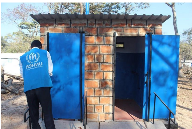
A newly constructed VIP toilet in Mantapala settlement ©UNHCR/Bruce Mulenga
