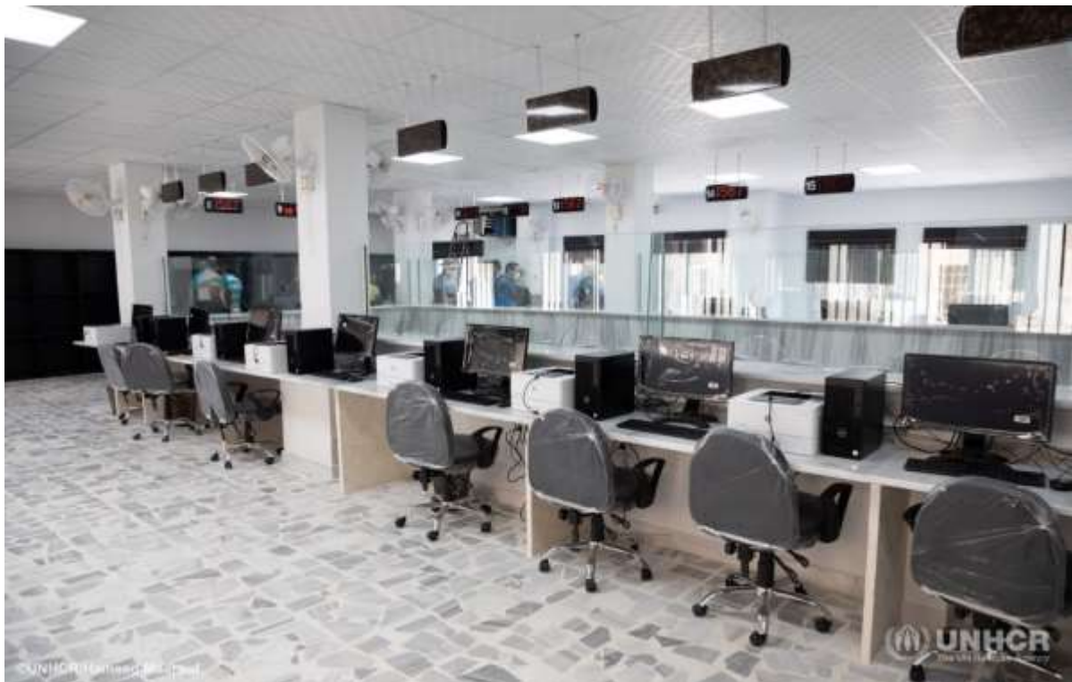
UNHCR and partners rehabilitated the civil registry office in the Old City, Aleppo. UNHCR/H. Maarouf.
