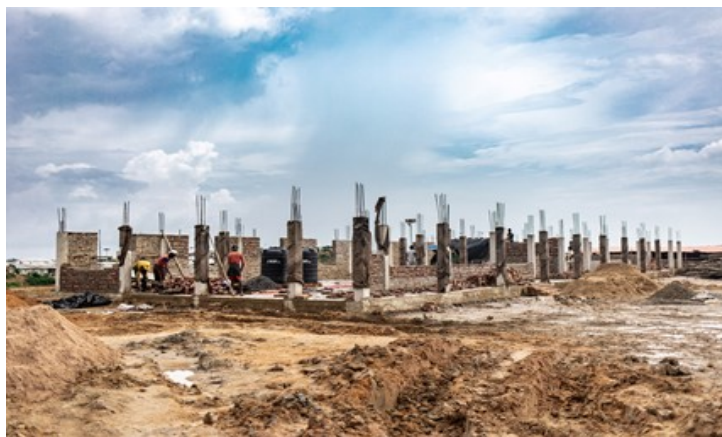
WFP E-voucher construction site, led by WFP's Engineering team
