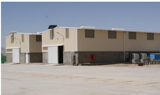
Humanitarian Response Facilities (HRF) in Quetta
