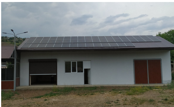
Collection centre powered by solar energy
