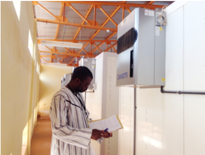
Adjustment of the refrigeration unit controller settings Credit: Adama Sawadogo
