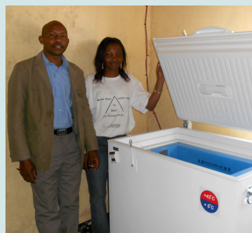
An SDD vaccine refrigerator installed at Pelewa dispensary in Kadijo, Kenya. Photo: Catherine Silali.
