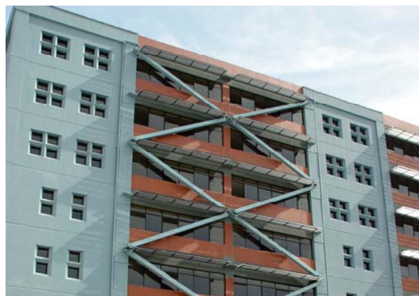
Structurally reinforced hospital, Ecuador (PAHO)
